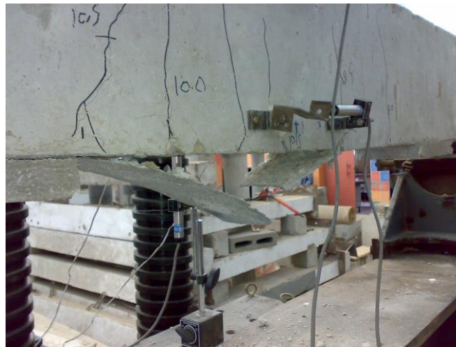
Fig. 15 : Failure mode of beams strengthened with CFRP
