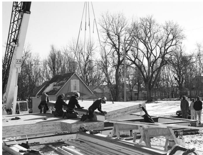
Fig. 5: Component Floor System.
