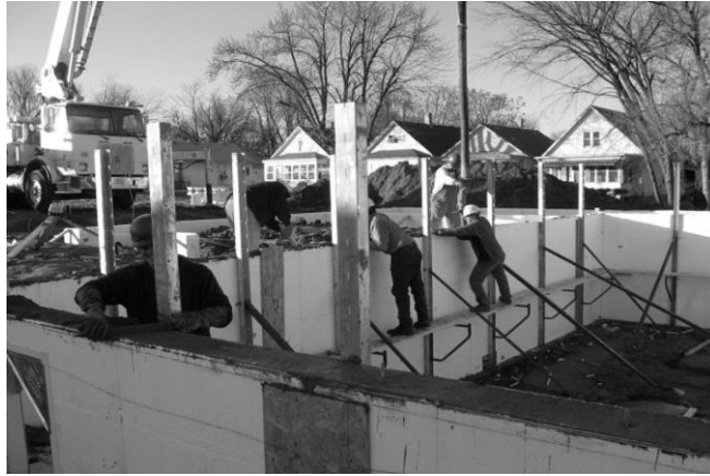
Fig. 4: Concrete Placement in Insulated Concrete Forms.
