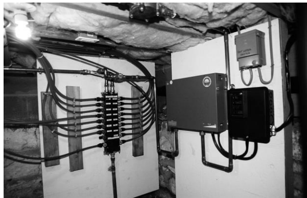
Fig. 6: PEX Plumbing Manifold
