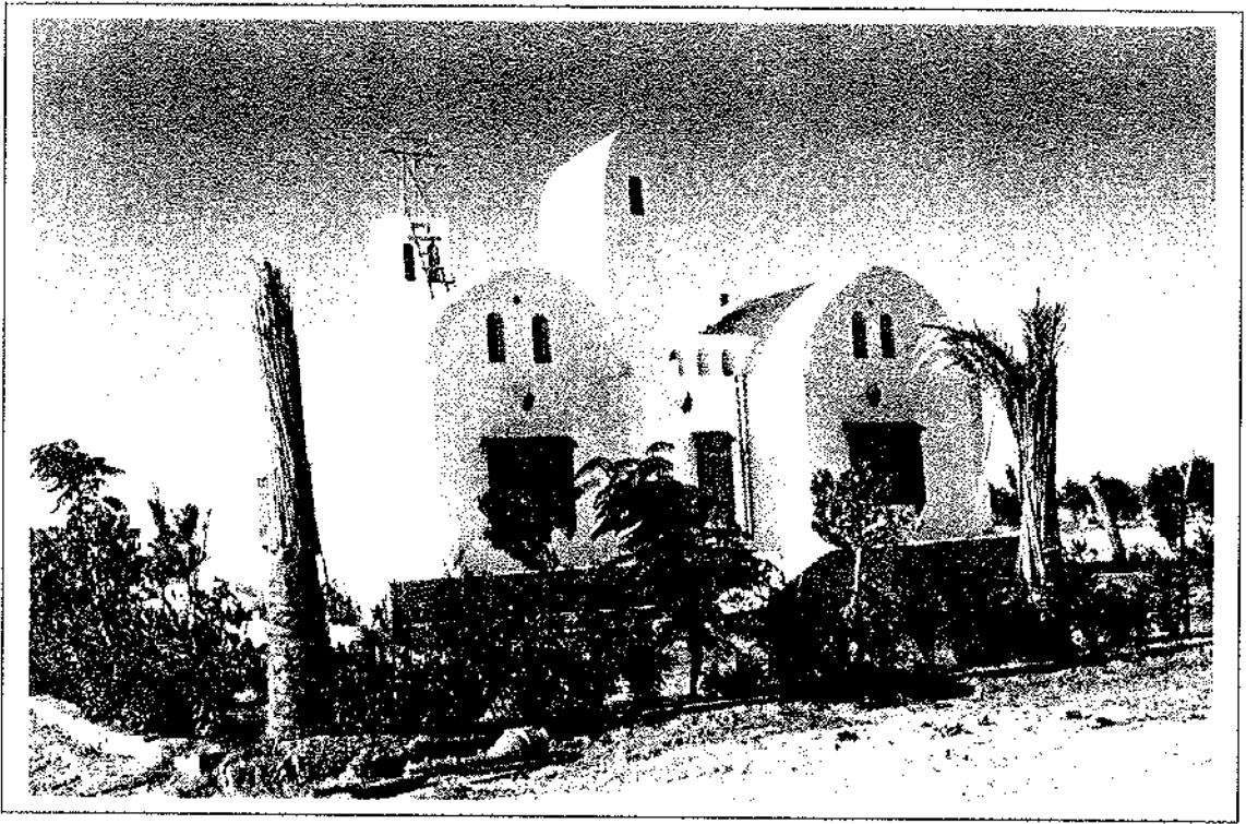
Figure 3a. Test House Built By HBRC In Toshky Region
