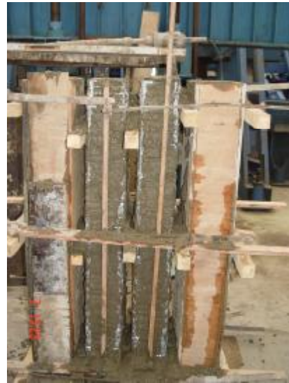
Photo 5: Casting of column specimens
