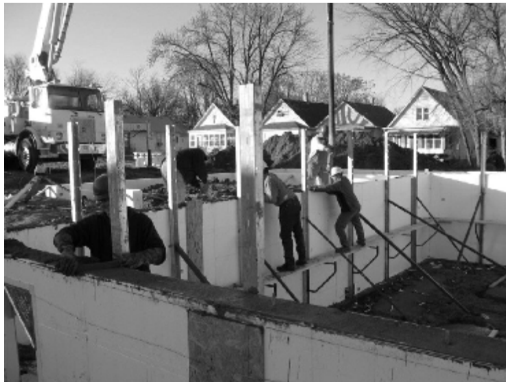
Fig. 4: Concrete Placement in Insulated Concrete Forms.
