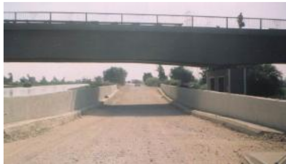
Fig. 11: Remedy Process of Kheneza Bridge
