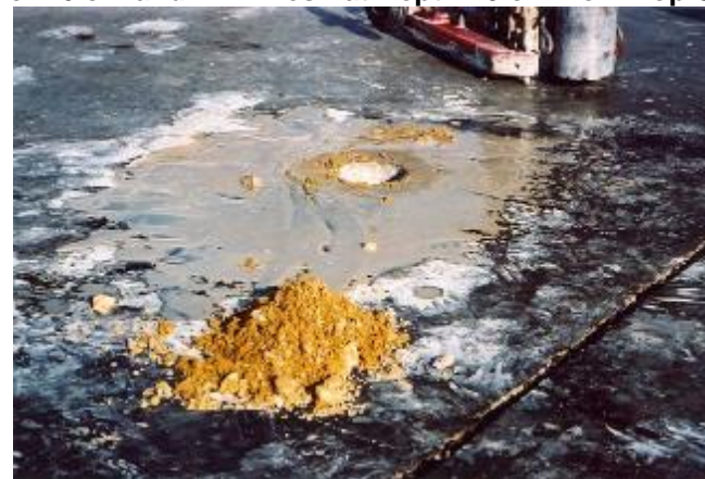
Fig. 12: Core Test Extended, in Depth, Through Base Material.
