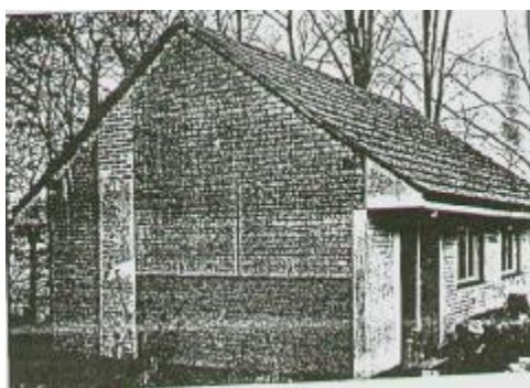
Fig 5: Experimental Building Constructed of Stabilized Soil at Garston [UK].
