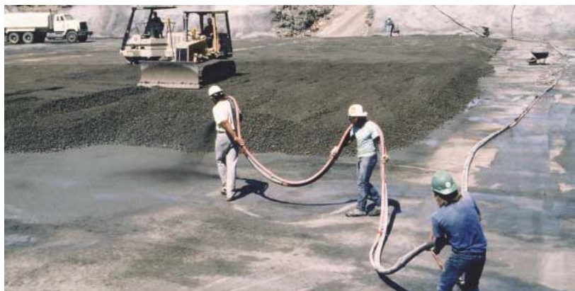
Fig. 1: Construction of Horizontal Joint [1]
