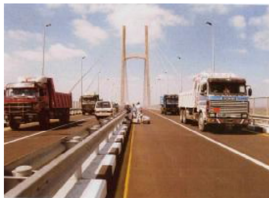
Fig. 16: Loading test of the Suez Canal Approach Bridge 40m span
